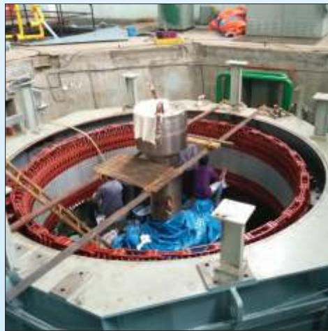
11.25MVA, 11KV Alternator Overhauling
