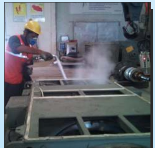
1MW, Stator Cryogenic Cleaning
