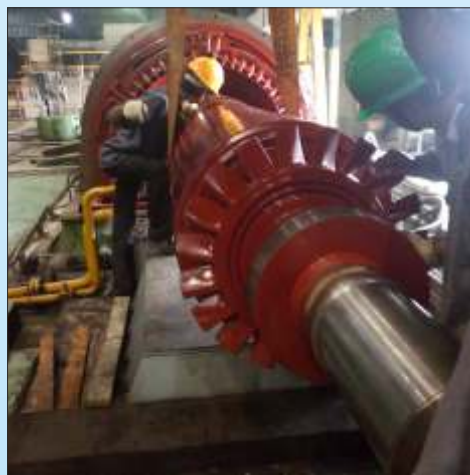
8MVA, Alternator Rotor Threading In
