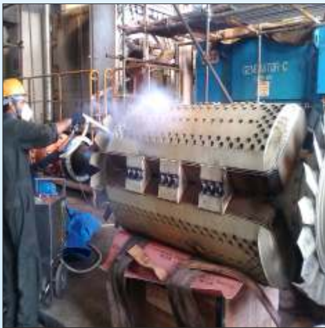
35MVA, Alternator Rotor Cryogenic Cleaning
