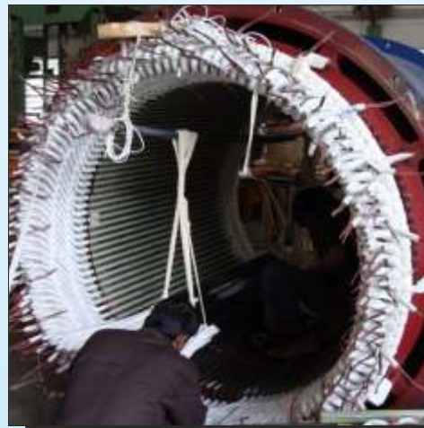
8MVA,11KV, Alternator Stator Rewinding
