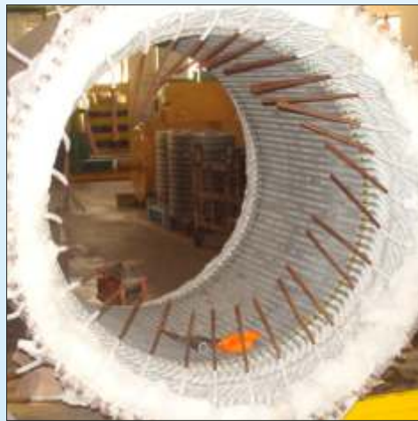
6MW, 6.6KV, Stator Rewinding
