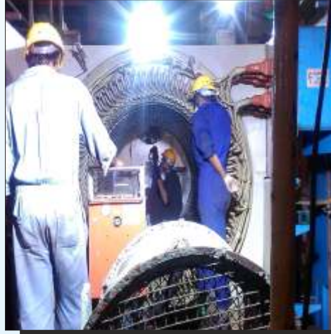
35 MVA, Stator, Cryogenic Cleaning
