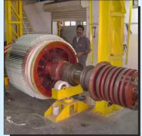
4MW, Slipring Rotor Rewinding
