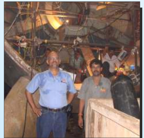
6MVA, 64 Pole Stator Rewinding Under Progress
