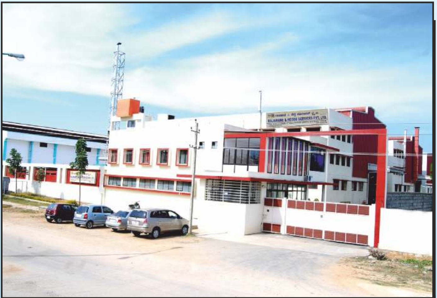
Major Repair Works at Tumakuru
